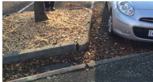
Difficulties in managing leaf litter as street sweepers cannot access gap between tree 'island' and kerb
