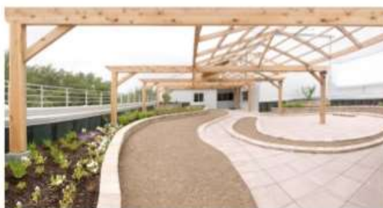
Green roof and permeable surfaces slow down and reduce rainfall runoff at a James Madison High School Agriscience Magnet Program building in San Antonio
